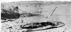
Figure 71. Another method to simulate an entrenchment is to place burlap or cloth in the outline desired and then fill in the simulated excavated portion with waste oil, paint, or scrapes of dark material. Note that the simulated parapet is formed by rolling under the edges of a large piece of burlap and creating the illusion of the mound of a parapet by piling sand under the burlap edges. The excavated portion of the slit trench is simulated in this figure by waste oil and dark colored salvage scraps.
